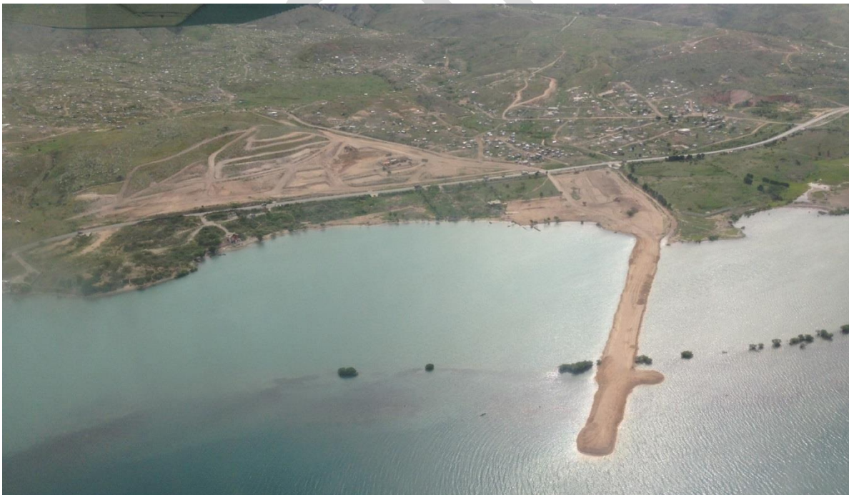
Figure 2 -Jetty Construction at July 2013
